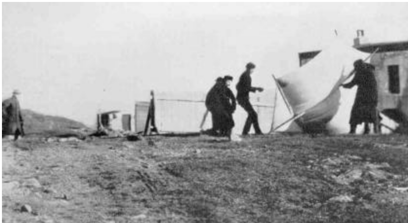
Figure 3. A scene from Signal Hill with the kite antenna being hoisted by Marconi and his support personnel. ( Newfoundland December 1901 )
